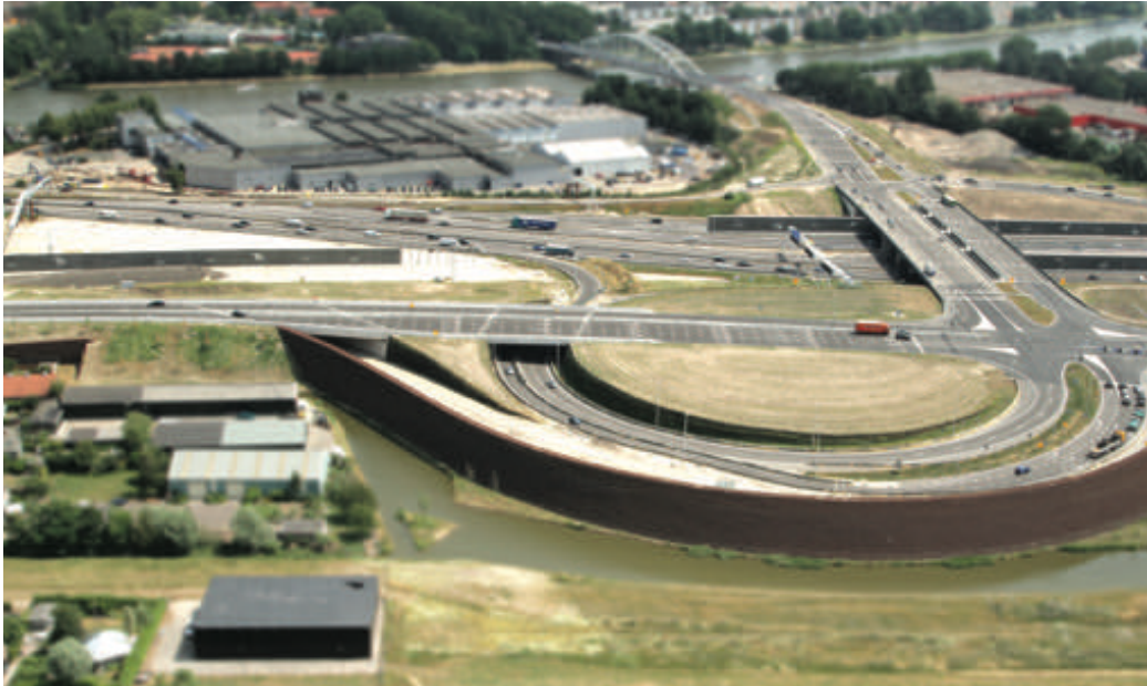
Figure 6 – Large scale geogrid-reinforced earth structures as sound barriers and soil retaining walls at highway junction A2 Hooggelegen Utrecht, The Netherlands.
